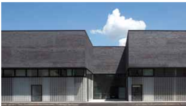
Top architect Botticini created the facade of the “Brescia Swimming Centre” using a total of 5,260 m 2 of clinker brick slips in “336 metallic black”.
