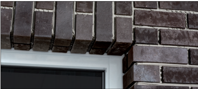
Window lintel perfectly replicated with angles.
